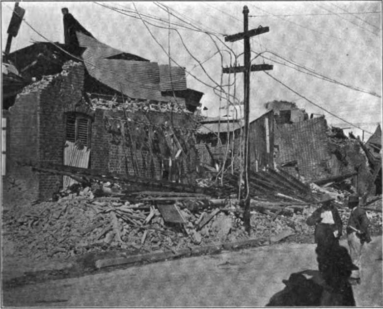
FIG. 13. View near the foot of East Street, Kingston, taken eight days after the earthquake of January 14, 1907, showing effect of the shock alone without fire. (The writer's laboratory was half a block from this, on the opposite side of the street.)
